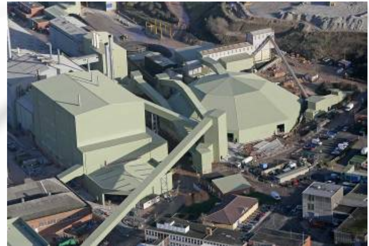
East Leake plant (UK) 2007
