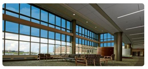
By reducing sunlight transmission while maintaining transparence, electrochromic glazing saves energy and enhances well-being for inhabitants
