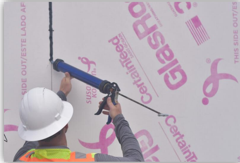
GlasRoc Sheathing is a lightweight, paperless gypsum board with a water-resistant core and fully embedded glass mat for exterior applications
