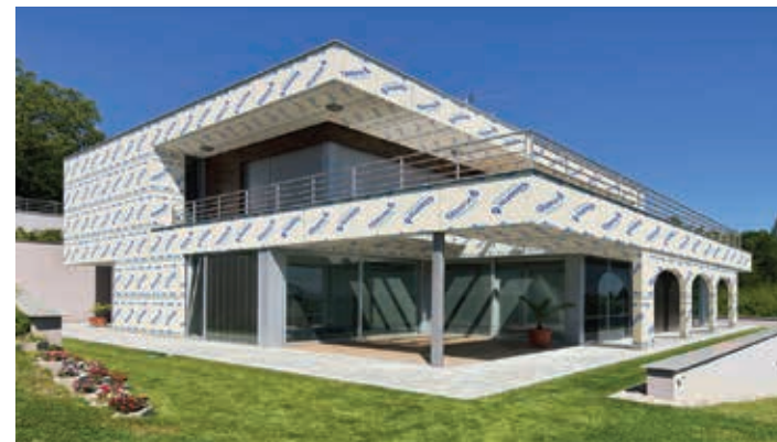
Glasroc X is a solution provided by Rigips , which combines an Adfors non-woven fleece with a Gyproc sheet and provides the benefits of protection against humidity, both inside and outside. This solution is supplemented by the application of mortars developed by Weber.
